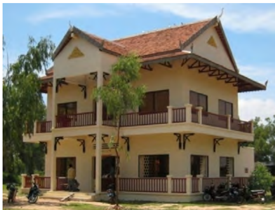
Prasat Bakong District Office
